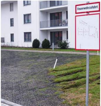
Whether it is a new installation or renovation of existing emergency access areas, if replanting is desired, the cover or soil builup can become a hazard. As a direct result, the surface loses its load-bearing capacity and can no longer withstand the demands placed on it by the fire department. This can hinder reaching the scene and put the safety of residents and rescue workers at risk.
