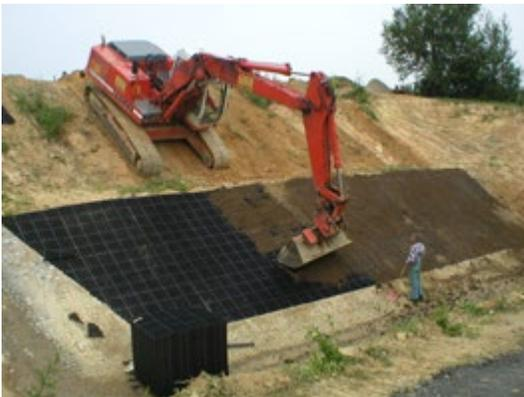
With over 200 expansion joints per square meter and 36 notched interlocking connectors per square meter the ECORASTER® counters the forces which are impacting the embankment. Erosion of the solum, soil destruction e.g. by rainwater made channels, line-shaped erosion and nutrient washout can be prevented by a proper installation of the ECORASTER® system.
